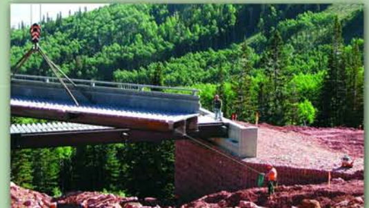
Installation of Pre-Assembled Beam Bridge
