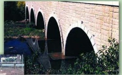
Multiple Arches with Concrete Headwall with Stone Form Liner
