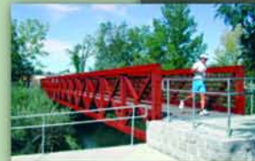
Double Diagonal Truss with Hardwood Deck
