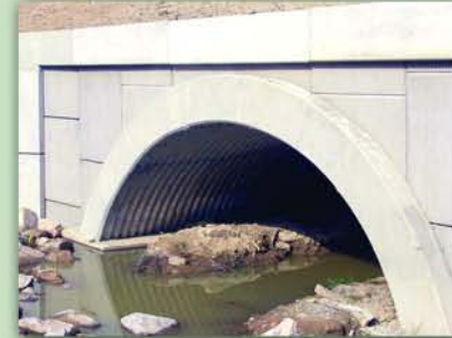
Multiple Arches with Concrete Headwall with Stone Form Liner
