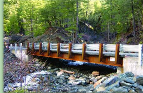
Weathering Steel Bridge
