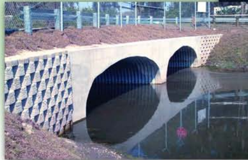
Twin Box Culvert with Concrete Headwall and Segmental Block Wingwalls
